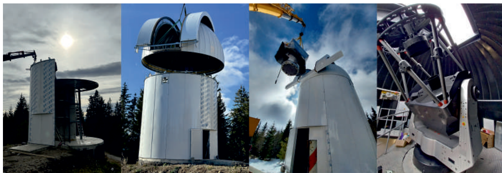
Fig. 1. The new dome and AZ1500 telescope
